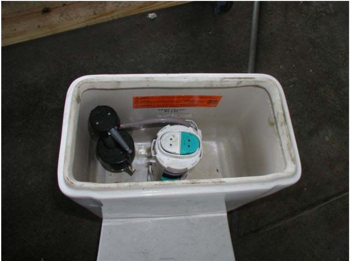
Figure 6: Dual-Cycle Water Closet
