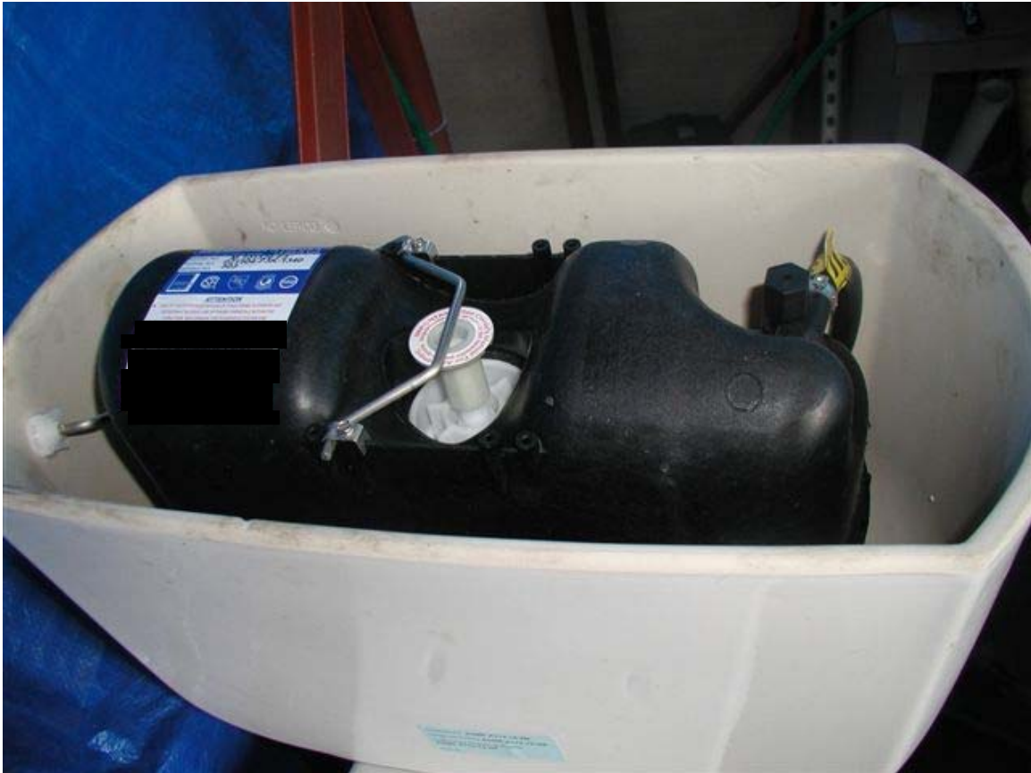
Figure 5: Tank of a Pressure Assisted Water Closet
