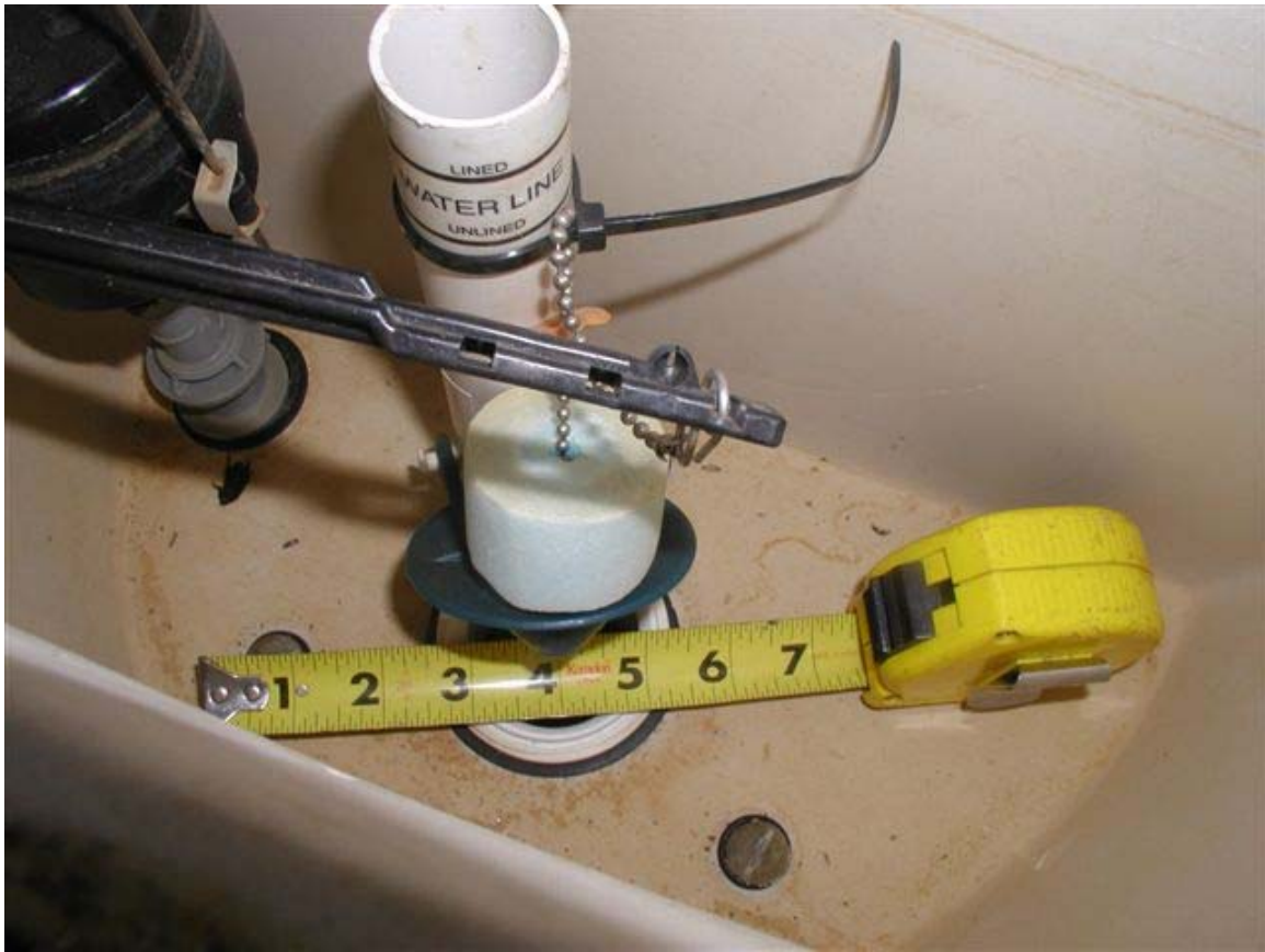
Figure 3: Tank of Typical “Standard” Siphon Water Closet
