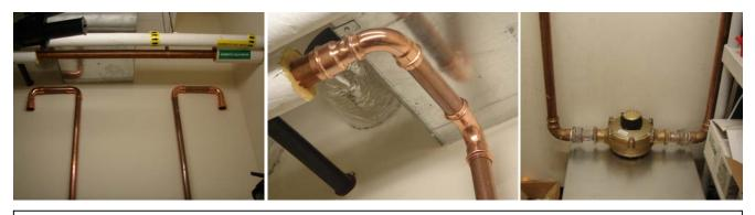
The above photographs show existing supply piping, piping modifications, and the new water meter.
