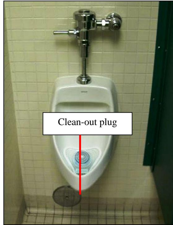
Figure 5. Clean-out plug example.
