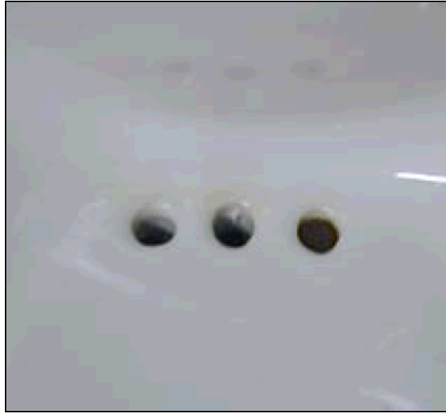
Figure 20. Drain holes in the bottom of the bowl in a Duravit non-water urinal.
