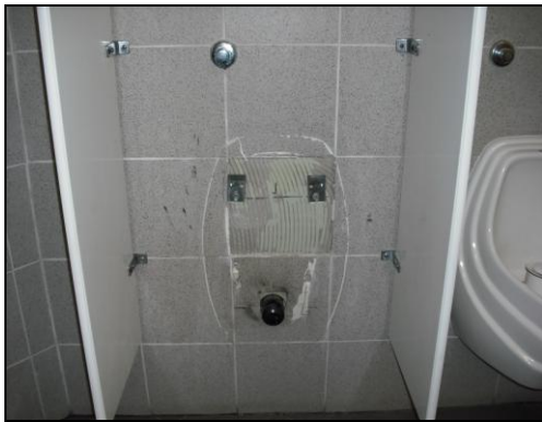
Figure 29. Non-water urinal removed September 2008 for pipe inspection.
