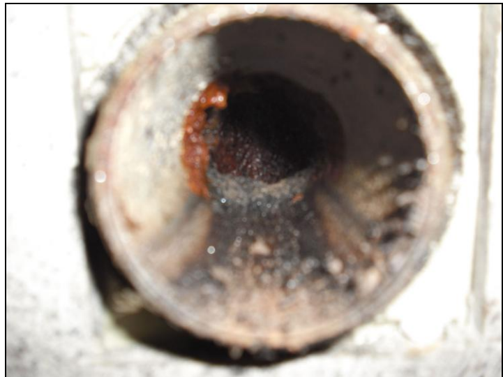
Figure 30. Close-up detail of the horizontal pipe nipple immediately after removing the non-water urinal, after six years of continuous operation.
