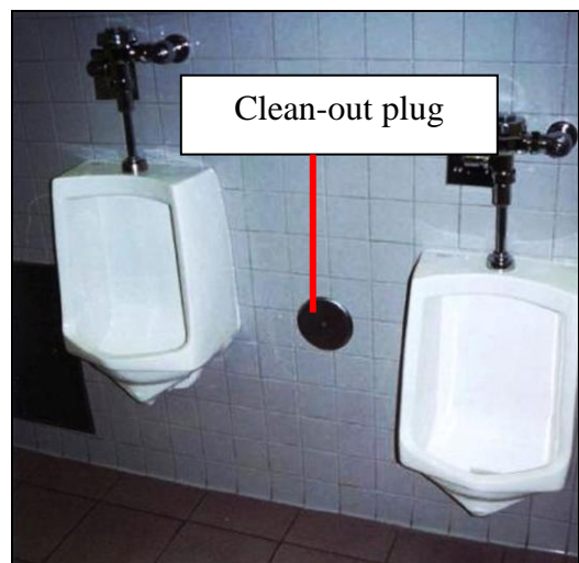
Figure 3. Clean-out plug example.
