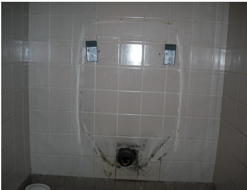
Figure 26. Non-water urinal removed in August 2008 for drain line inspection.
