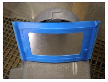
The toilet dam device is essentially a method of blocking off a section of the toilet tank and creating, in essence, a smaller tank. By blocking off one side of the side you reduce the volume of water that it takes to fill the tank.
